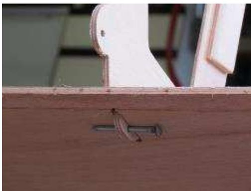
Panels are clipped into place using the tab and slot method and held in position by sliding a nail through a predrilled hole in the tab.
