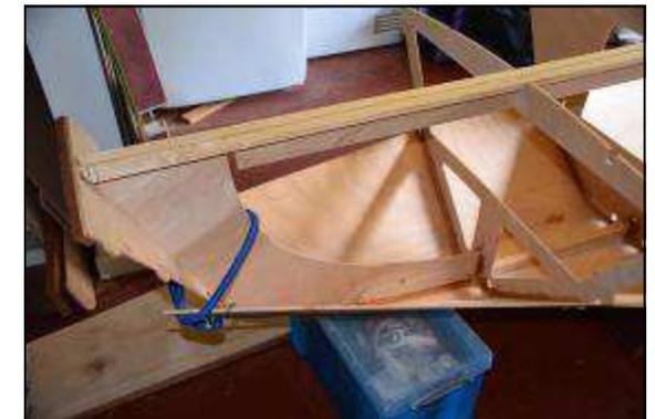
Panels are wired together to ensure a close fit, but these wires are later removed after the boat is spot welded using epoxy (John's good idea so you don't see the wires in the finished product—the building instructions say to tape over them)
