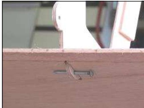
Panels are clipped into place using the tab and slot method and held in position by sliding a nail through a predrilled hole in the tab
